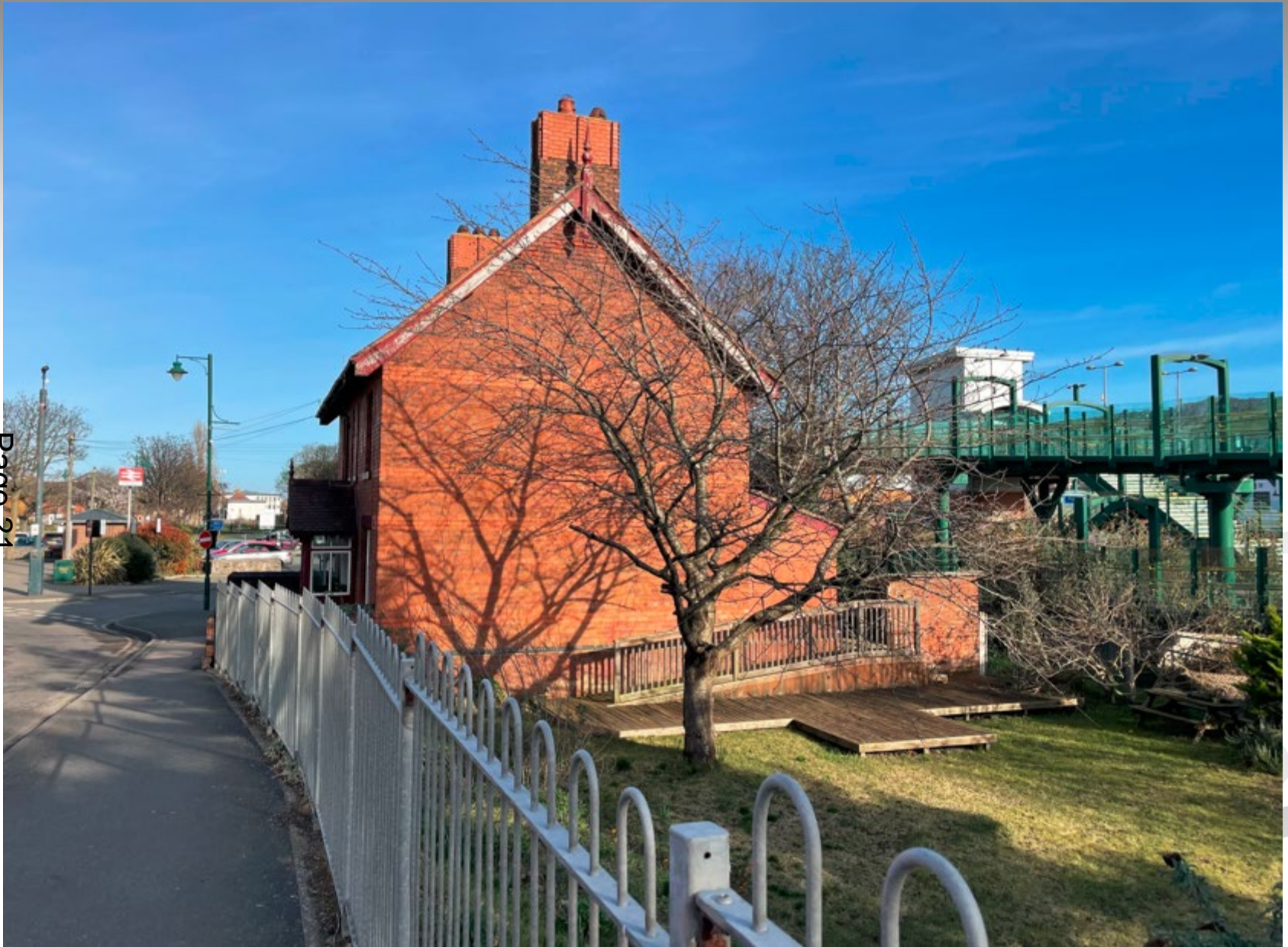
View of site from Bridge Road (West Side)
